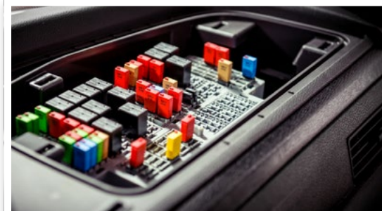
In-cab electrical panel
